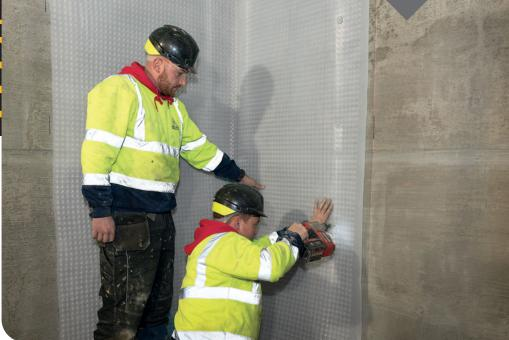
They ensure a water tight application of the Wykamol Cavity Drain Membrane Systems. Wykamol Plaster plugs are of a high quality and can be used in a range of applications and on multiple substrate types. The tailor made Thermoplastic Elastomer seal ensures application of the membrane is water tight.
