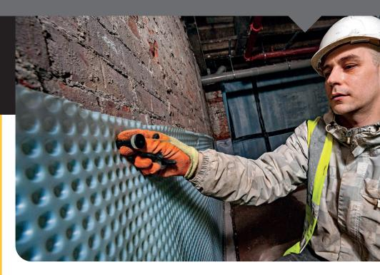
They ensure a water tight application of the Wykamol Cavity Drain Membrane Systems. Wykamol Brick plugs are of a high quality and can be used in a range of applications and on multiple substrate types. The tailor made Thermoplastic Elastomer seal ensures application of the membrane is water tight.
