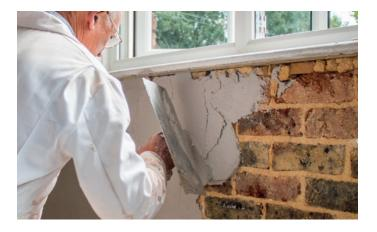
Any other finishing is carried out once the curing process is complete, after at least 14 days. Redecorate using a non-vinyl based emulsion paint.
